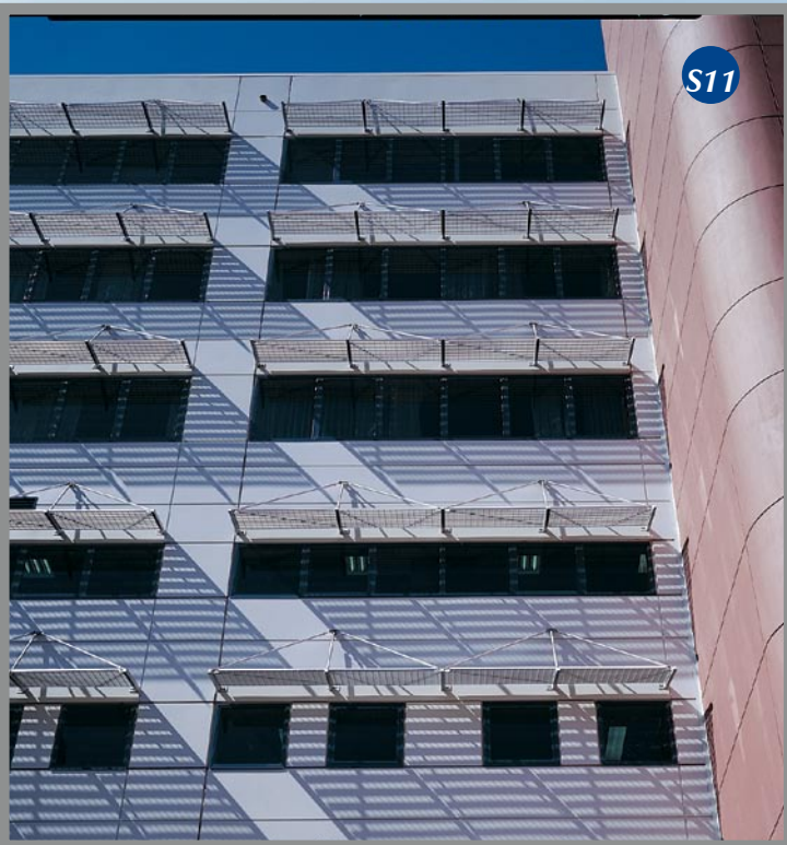
Prince of Wales Hospital, Randwick, NSW, SS203/60 louvre with RHS and CHS support framing, suspended from cast-in ferrules inside the GFRC façade.
